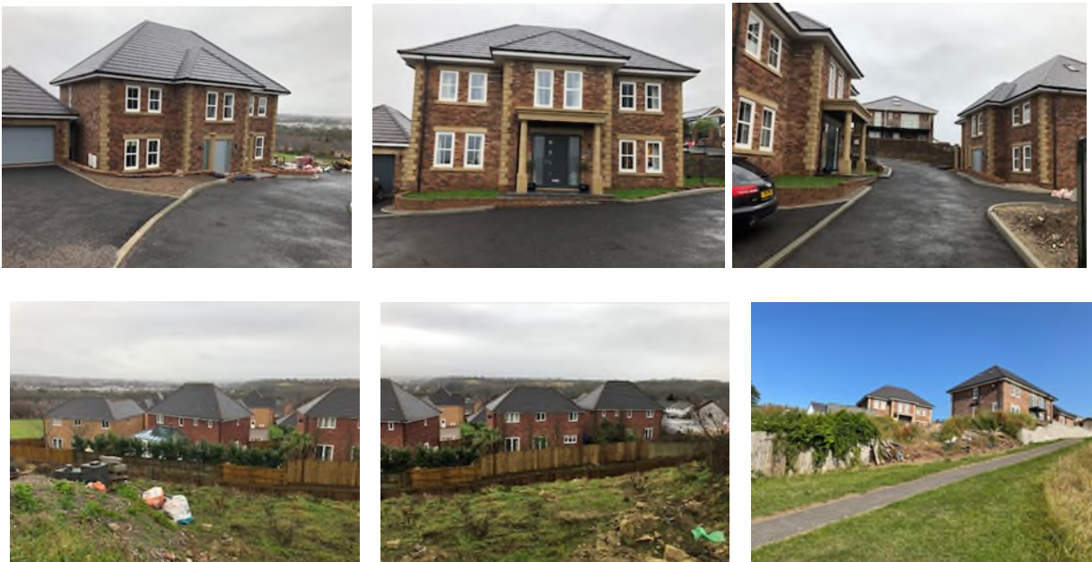
Fig. 5 – Photographs of the application site
